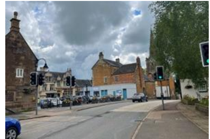
Constrained road space with high traffic volumes forms a critical junction at A6003 Ayston Rd, North St, and A6003 Orange St at a key pedestrian and cycle gateway to Uppingham town centre.
