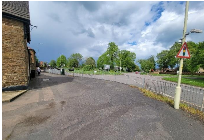
Wide junction corner radii and cluttered junction crossing arrangements at B668 Burley Rd/ Ashwell Rd – this critical junction is a key link between Oakham School sites.
