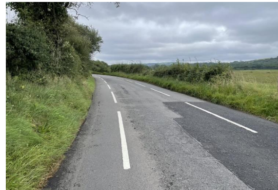
More open rural roads with low traffic can benefit from centre line removal and the addition of advisory cycle lanes
